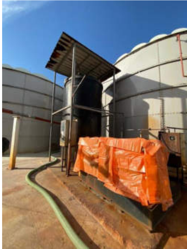
Figure 6: Ferric Chloride storage tank
